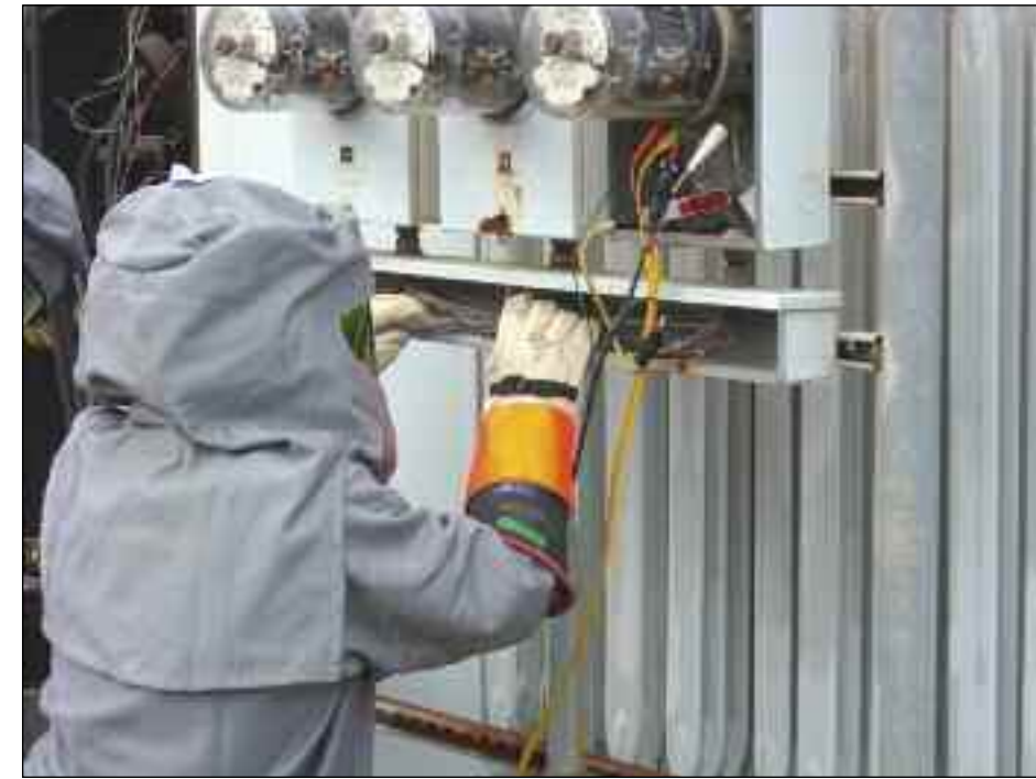
Metering of NAS facilities will continue into 2010.
